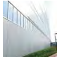
Exterior wall with photocatalytic coating
